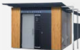
Vertical open-work natural wood cladding (Douglas Pine)
