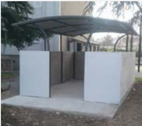
Centu'Park Specific finishing
